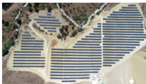
Green Energy Group Project Ayios Ioannis Maloundas, Nicosia District
